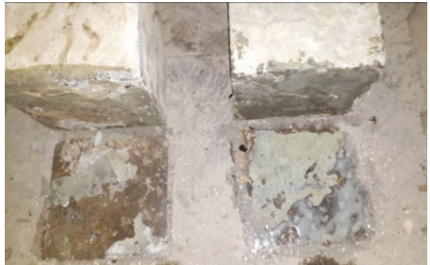
Fig. 18: Failure of the Bonded Plane in Horizontal Shear Test at Ultimate Load, for the case of Epoxy-Bonded Plane
