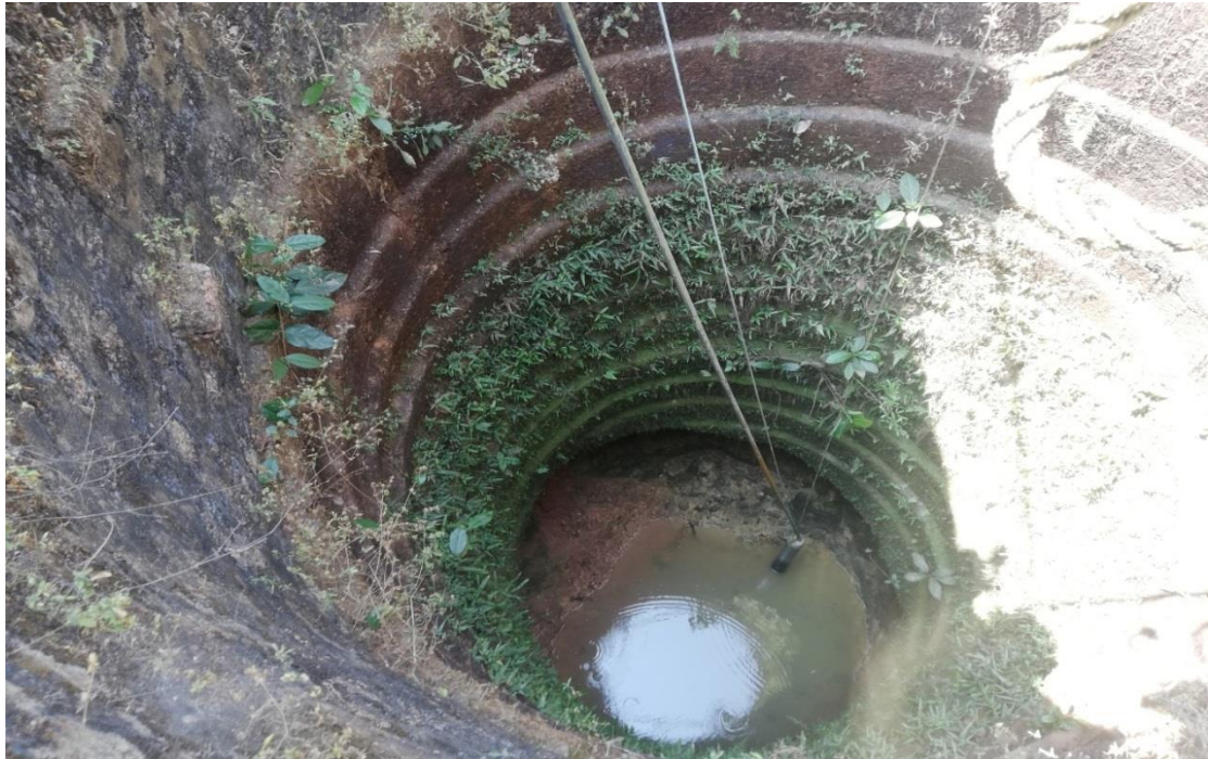
Fig. 4.5. Well No 8 with huge opening or caving at the bottom.
